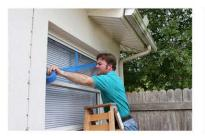
**REALITY:** Taping does not prevent windows from breaking, nor does it make them any more resistant to breakage. At a minimum, window shutters need to be made of 5/8" plywood or metal and fastened correctly in order to provide protection. Tested and approved shutters are always best.
